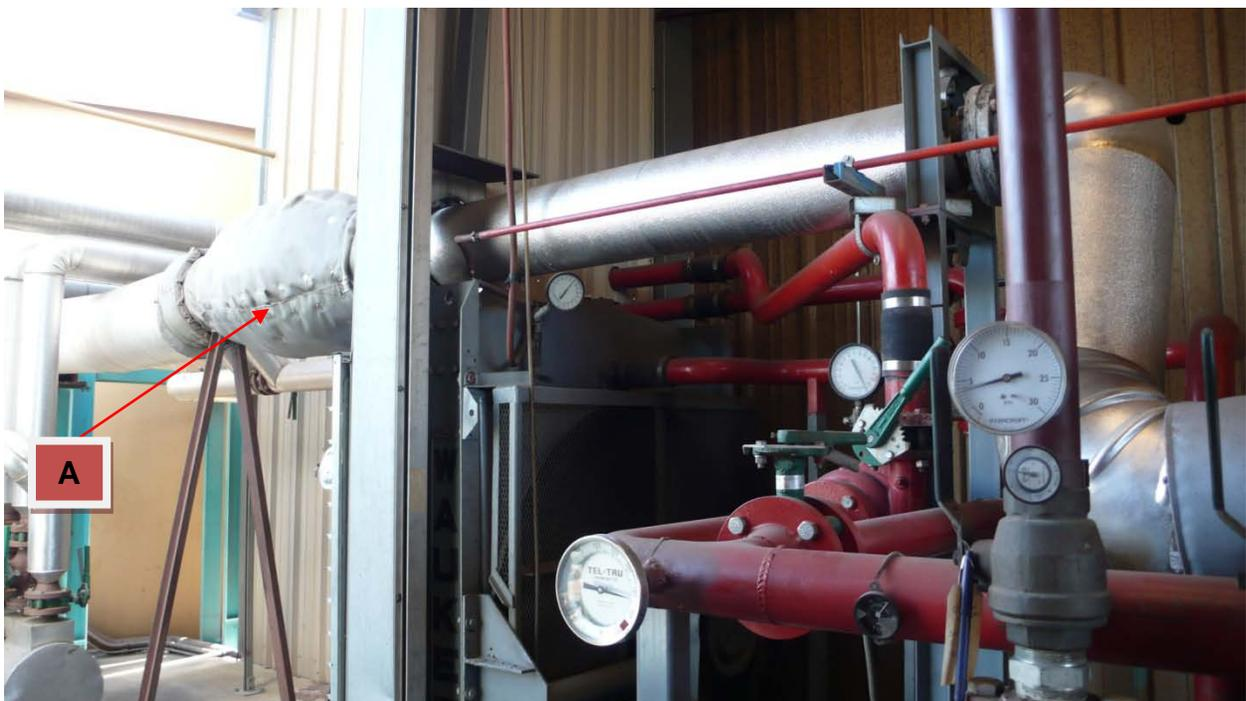
**Figure 7: Original exhaust piping viewed from engine toward catalyst (A).**
