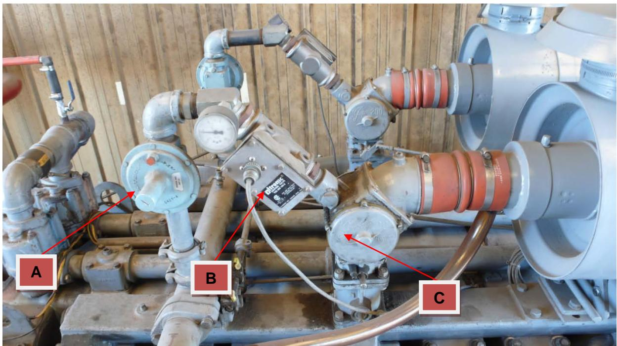
Figure 3: Regulators (A), solenoid operated gas control valves (B) and Impco Carburetors (C)
