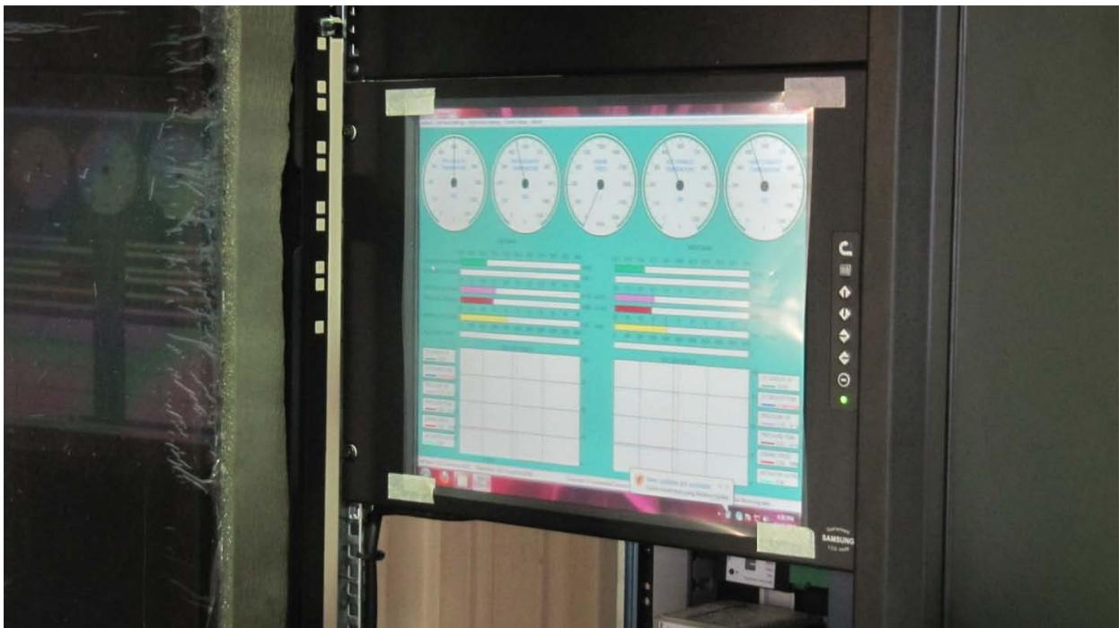
**Figure 13: Large, flat panel display allows monitoring of the position, settings and inputs to both valves. The software also logs data for later retrieval and analysis if needed. Data is presented numerically as well as graphically via dials, bar charts and a strip-chart like display**
